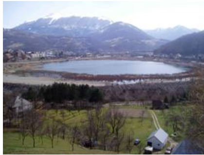
Tailing Dam, Mojkovac Mine, Serbia and Montenegro
