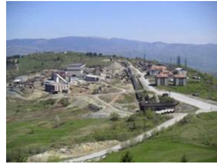
Rosia Poieni smelter, Romania
